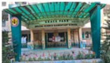
The PAGCOR Building which is intended for Special Science Elementary School.
